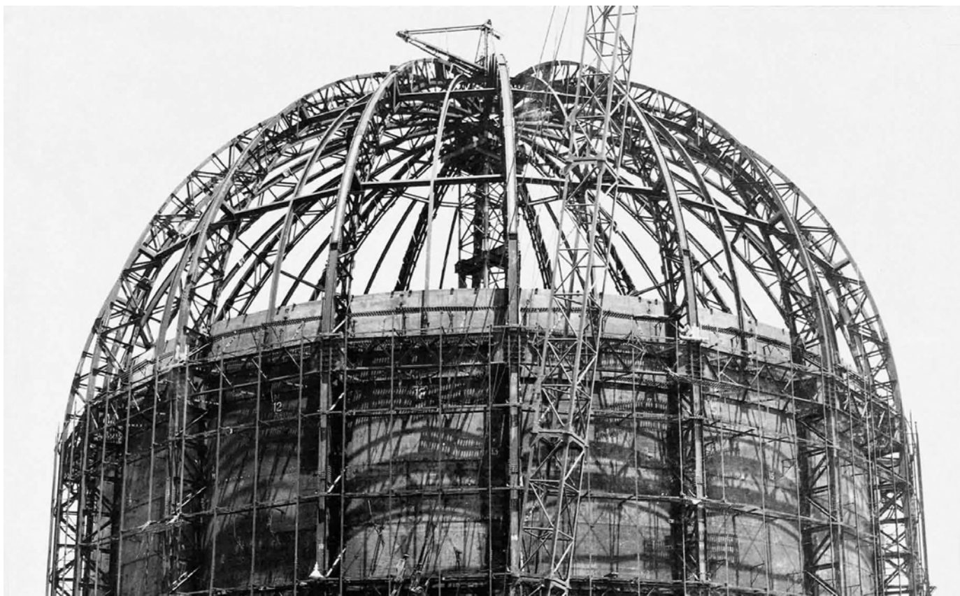
The Bhabha Atomic Research Centre (BARC) under construction at Trombay (1957 to 1961)
